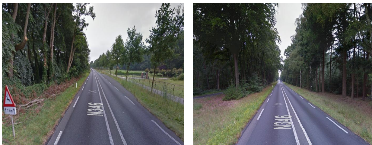
Figure c2. Street view of the N346 at hmp 6.1 (left) and hmp 10.0 (right) (googlemaps.com, 2014)
