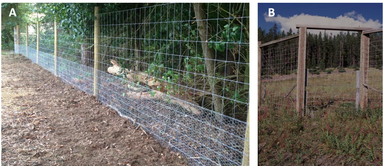
Figure 21: A) Fencing for deer and B) a one-way gate in case a deer accidentally ends up at the wrong side (e.g. roadside) of the fence (Derbyshire Stock Fencing LTD, 2014 and Huijser et al. , 2008 respectively)
